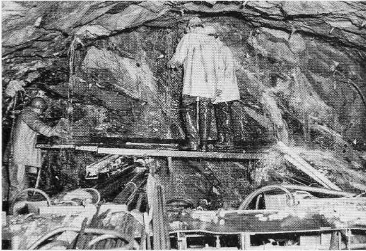
Drilling from jumbo in tunnel
