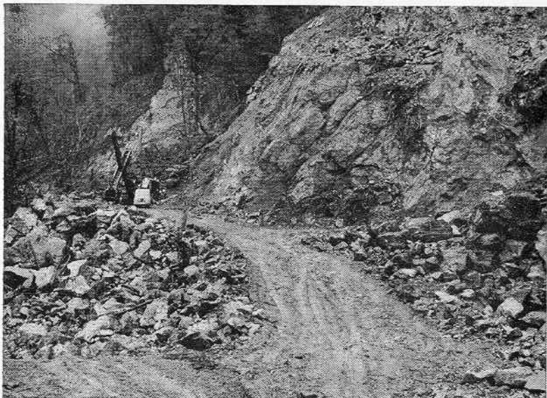
Early construction of Wilmot Pass road in summer
