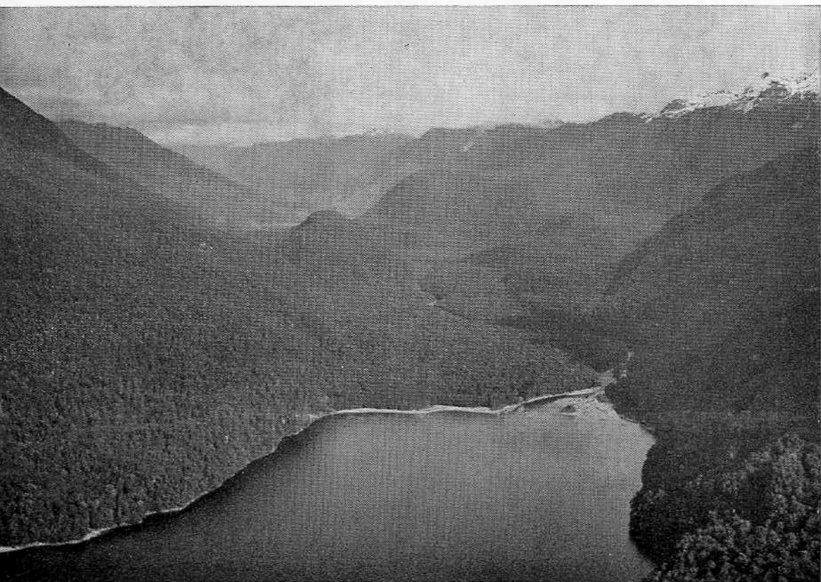
Early view of South Arm, Lake Manapouri, showing Grebe Valley which the transmission line will follow. South Arm camp site is now built on right bank of Grebe River
