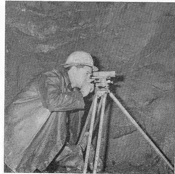
Surveyor sighting in tunnel to ensure correct alignment
