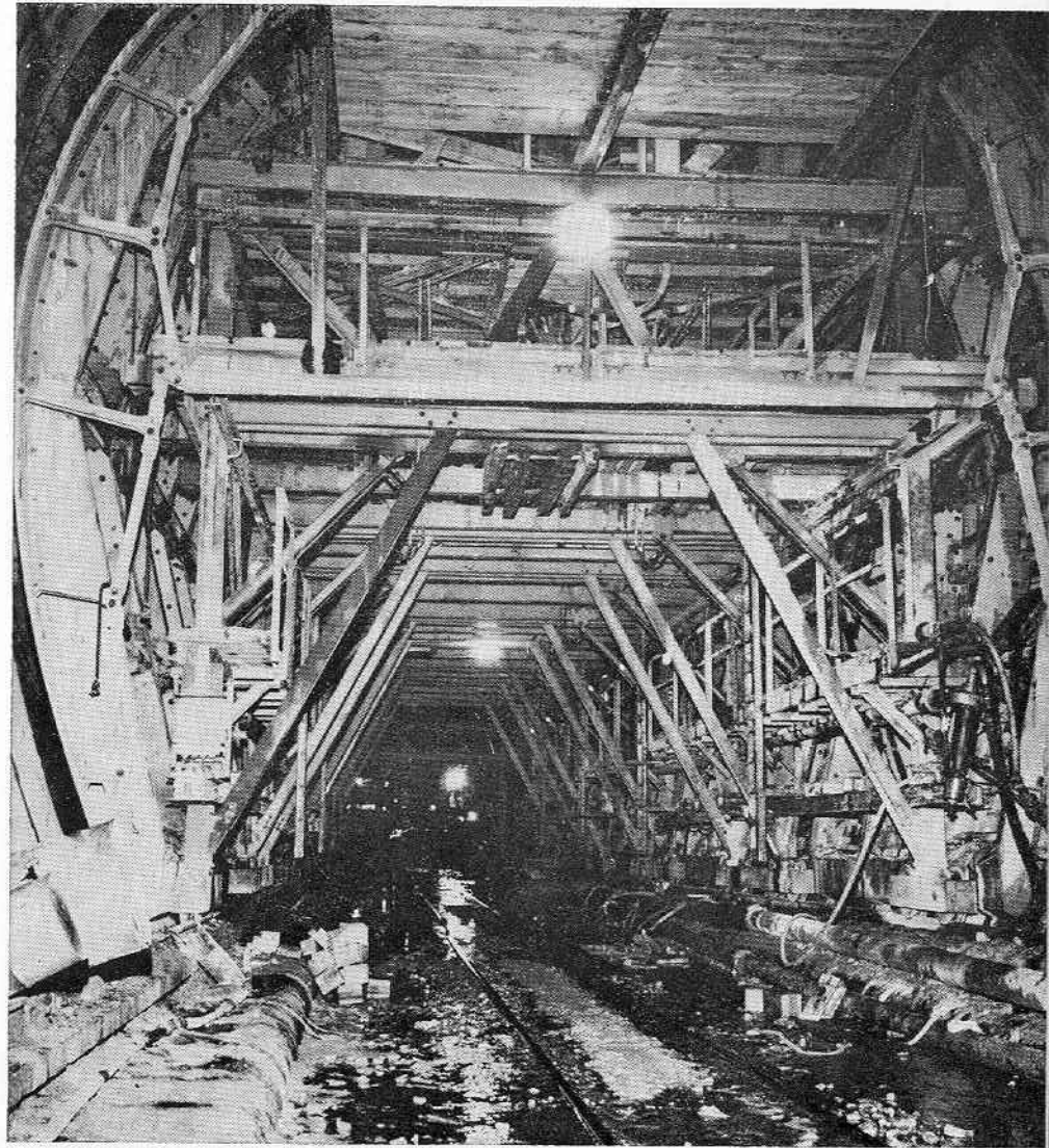
Formwork in the 6 mile, 30-ft-high, tailrace tunnel
