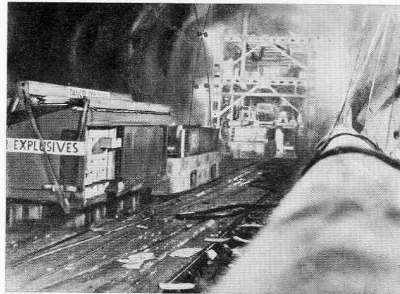
Explosive truck at face of working
