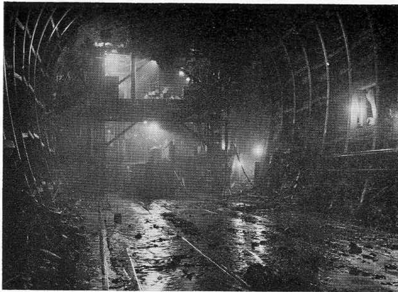
Drilling jumbo, No. 3, tailrace tunnel, Deep Cove
