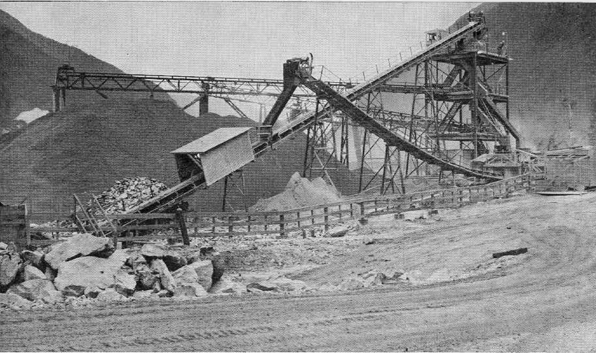
Concrete aggregate plant at servicing area, Deep Cove
